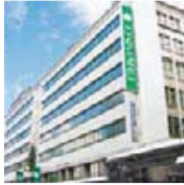
Daimaru Kyoto (Floor space: 50,830 m 2 )
