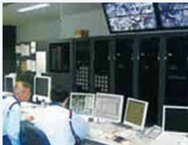
At the disaster prevention center of Daimaru Tokyo store, we have centralized control through various monitors to confirm the safety of the whole building.
