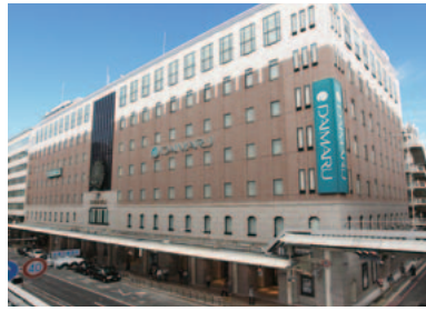
Daimaru Kyoto (Floor space: 50,830m 2 )
