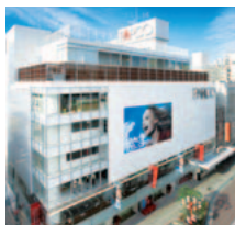
Shizuoka Parco 6-7, Koyamachi, Aoi-ku, Shizuoka B1F-8F Opened: March 15, 2007 www.parco-shizuoka.com
