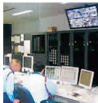
At the disaster prevention center of Daimaru Tokyo store, we centralize control through various monitors to confirm the safety of the whole building.
