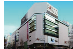
Sapporo PARCO 3-3, Minami 1-jo Nishi, Chuo-ku, Sapporo, Hokkaido Main Building: B1F-9F B2F-8F Opened: August 24, 1975
