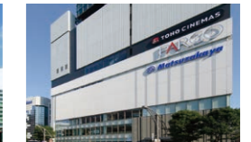
PARCO_ya Ueno 3-24-6, Ueno, Taito-ku, Tokyo 1F-6F Opened: November 4, 2017 Ueno Frontier Tower B1F, 7F-10F
