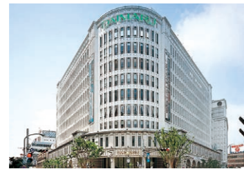
Daimaru Kobe (Floor space: 50,656m 2 )
