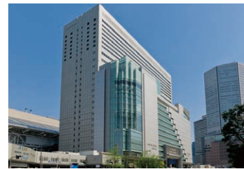
Daimaru Osaka Umeda (Floor space: 64,000m 2 )
