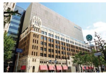
Daimaru Osaka Shinsaibashi (Floor space: 46,490m 2 )
