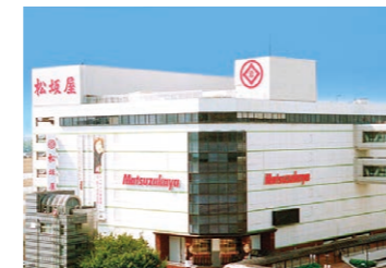
Matsuzakaya Toyota (Floor space: 18,220m 2 )
