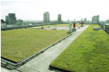
Daimaru Shinsaibashi Rooftop
